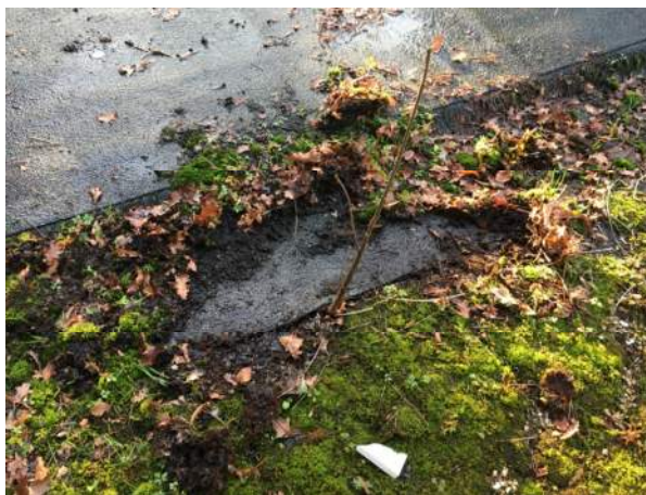
Organic growth from within the weather proofing, should be removed as part of a maintenance programme.
