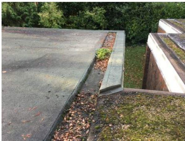
Channel for RA 3 blocked as is outlet. A maintenance schedule should be adopted to keep drainage clear.
