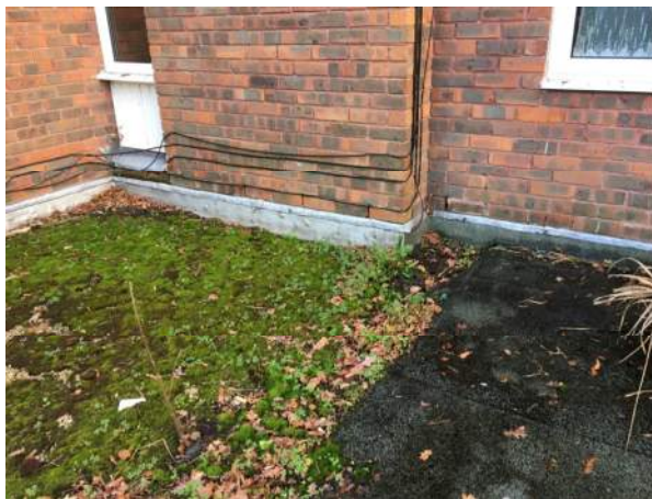
Change in height dividing car park roof RA4. Minimal covering of lead flashing. Cavity trays/DPC will need raising
