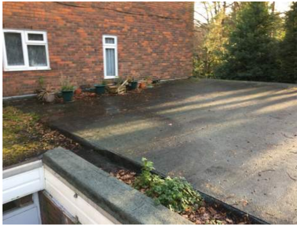
Good falls to a blocked channel in the foreground. Upstand height at far perimeter is below 50mm . Mineral felt is weathered and aged.
