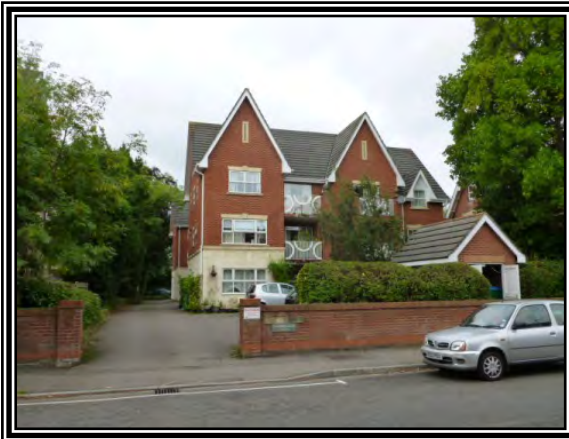
Twyford House, 15 Hulse Road, Southampton, SO15
