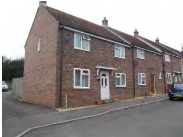
Gundry Road, Bridport
