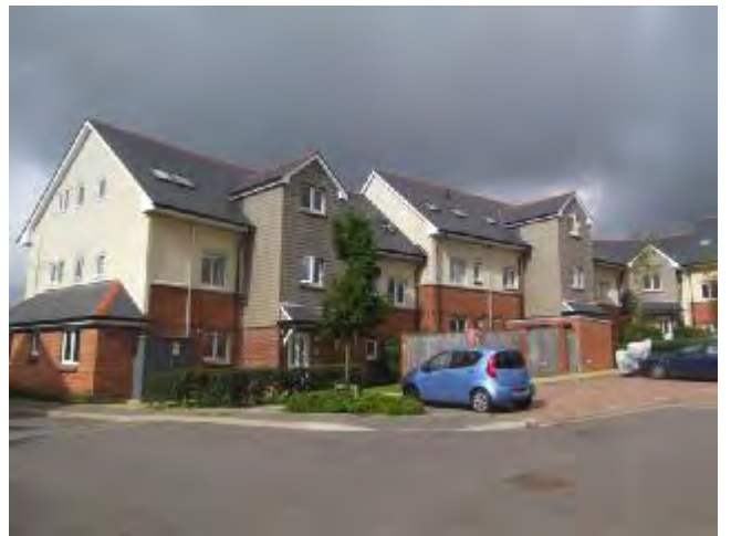
Holzwickede Court, Louviers Road, Weymouth
