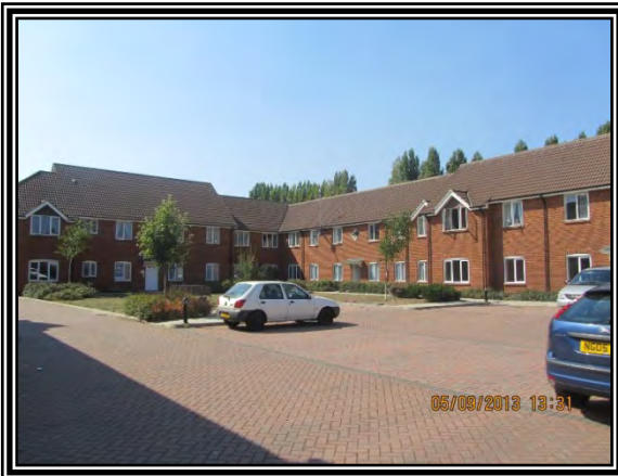
Ashdown Court, Bath Road, Padworth, Reading, RG7
