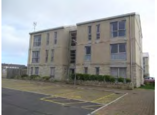
Lancriage Court, 39 Barleycroft Road, Portland
