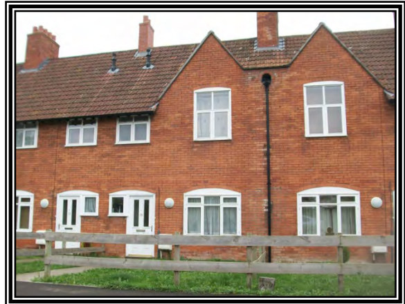
Beckbury Cottages, Old Beckbury Road, Glastonbury, BA6
